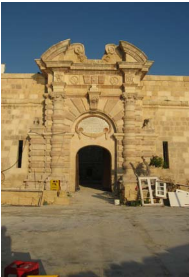
Figure 15. View of the recently restored Main Gate elevation
