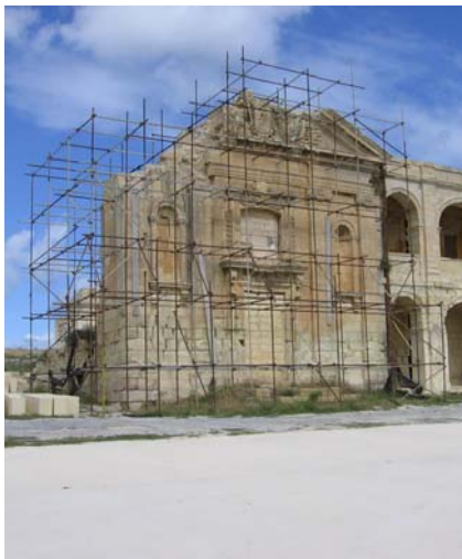
Figure 21. The chapel prior restoration
