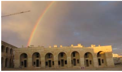
Figure 17. Barrack Block B
